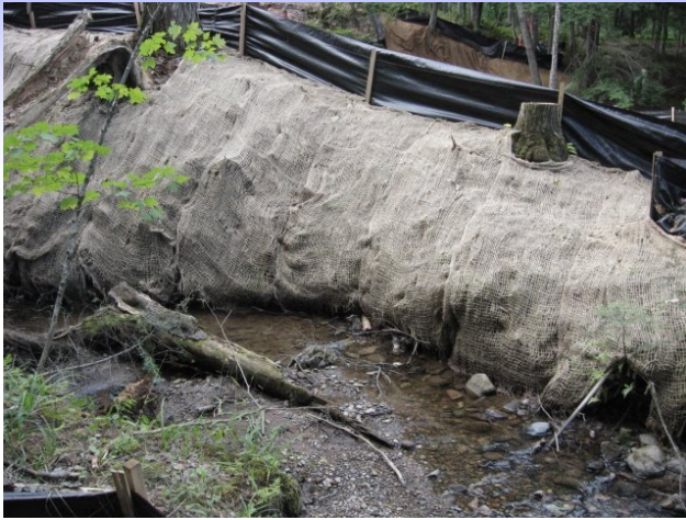
The sides of all slopes draining to the stream were polymer enhanced soft armored using APS 712 Silt Stop Powder.
