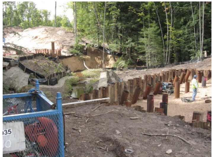
This is the beginning of bridge construction over a stream draining to the Salmon Trout River.
