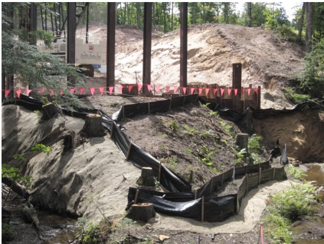
Polymer enhanced soft armoring and Sediment Retention Barriers were installed at the bottom of the slopes adjacent to the stream.
