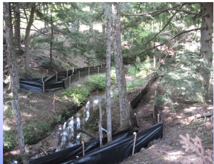
Sediment retention barriers (SRBs) were installed at the bottom of the slopes adjacent to the stream.
