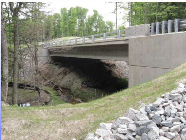
Construction of bridge finished with sediment contained on site and the stream was not impacted.
